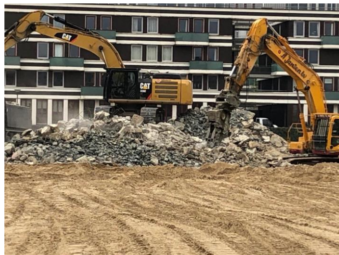
Figure 2: In-situ demolition waste treatment in the Netherlands (Den Bosch, April 2021)
