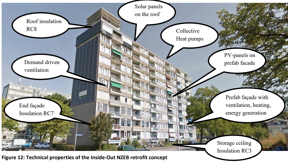
Figure 12: Technical properties of the Inside-Out NZEB retrofit concept
