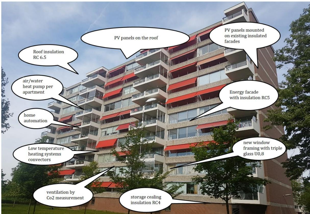
**Figure 14: Overview of the Happy Balance concept (adapted from Happy Balance, 2017)**
